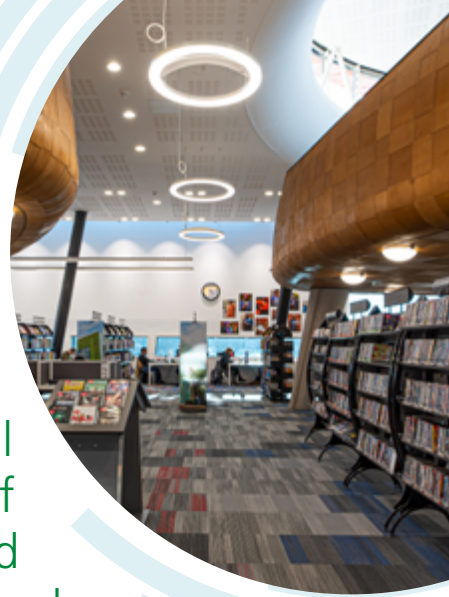
New LED lighting at Peckham Library
